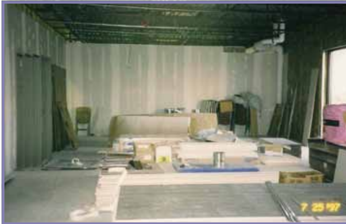
A classroom is in the process of being finished out in 1997.
